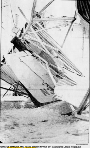
RUNS OF HANGAR AND PLANE SHOW IMPACT OF MAMMOTH LAKEE TREMBOR. The sturdy metal structure crashed inward with a loss estimated at $450,000.
